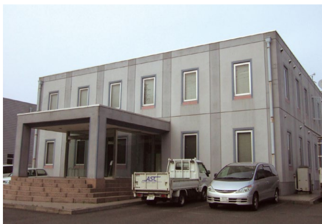
ACR Aikawa Office (Aiko district, Kanagawa, Japan)
